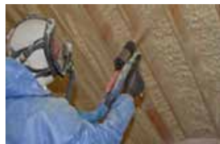
Image of 1" min. FILL method
